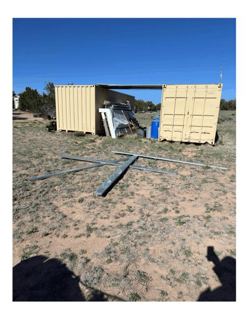
[Here you can see the two containers with the metal slats lying across the top between the containers, and see what was formed by a "dirt devil."]
